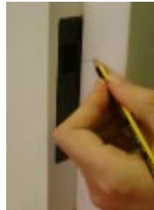
**Tip** Location of the bolt across the width of the door frame will vary due to the design of each door frame. Measure the distance from the recess to the door edge that closes first, then add 1-2mm to ensure that the bolt will sit in the recess comfortably. Measure this distance from the door jamb in the frame and mark it to provide a guide as to where to locate the bolt.
